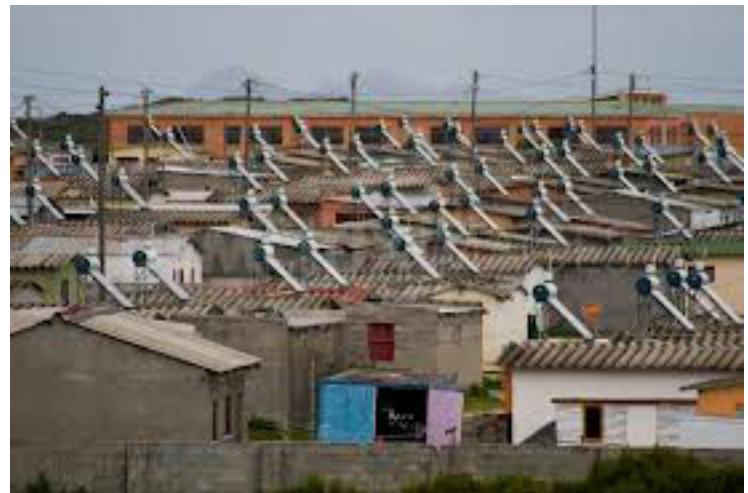
Left: Solar panel, North Africa; right: Solar heating, Cape Town
